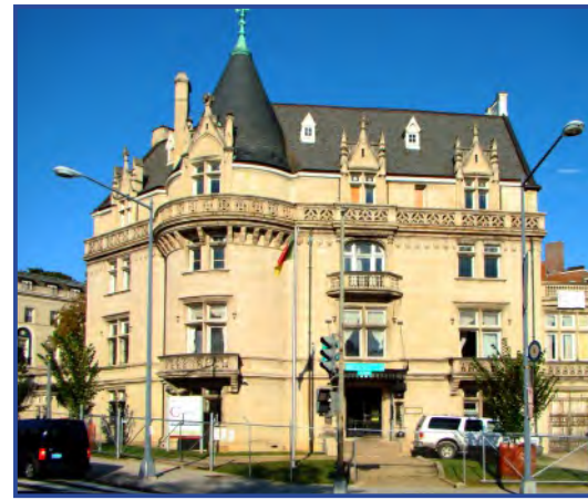
Building of the former Czechoslovak embassy (at 2349 Massachusetts Avenue), in which Vladimír S. Hurban served from 1936 as envoy to the United States, and since 1943 continued as ambassador. He was replaced by another well-known Slovak Juraj Slávik Neresnický in June 1946. Slávik stayed in office until March 1948, when he resigned in protest of Communist coup in his country and remained to live in exile.
