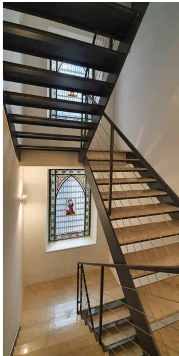
The building of the Permanent Representation of the Slovak Republic to the Council of Europe in Strasbourg following renovation. Detail of the staircase, right. (2018)
